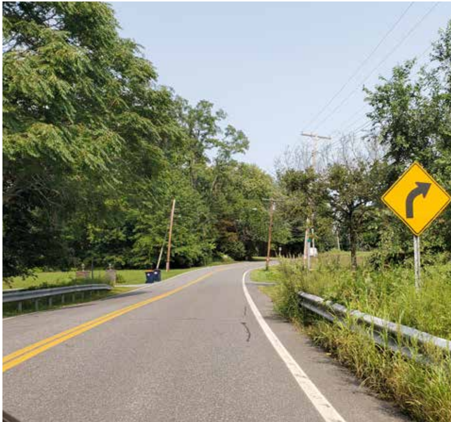
Rhinecliff Road culvert (photo facing north - cross-section location C)
