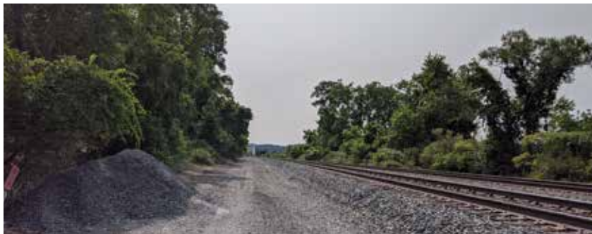
Rail corridor with space for an adjacent shared use path (photo facing south)
