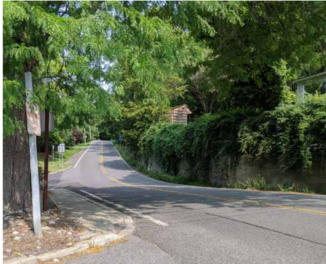
Existing sidewalk on west side and existing retaining wall on the east side of Charles Street (photo facing north - cross-section location A)
