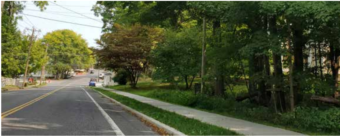
Existing sidewalk on south side of W Market Street (photo facing east)
