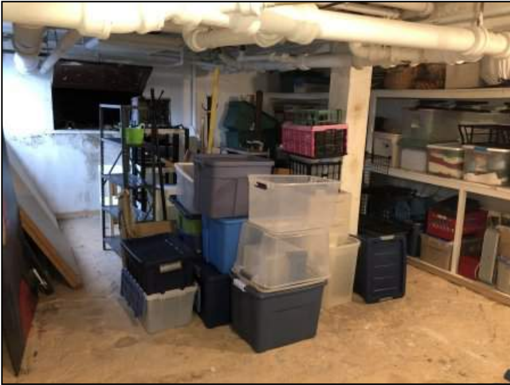
Storage room in basement (2)
