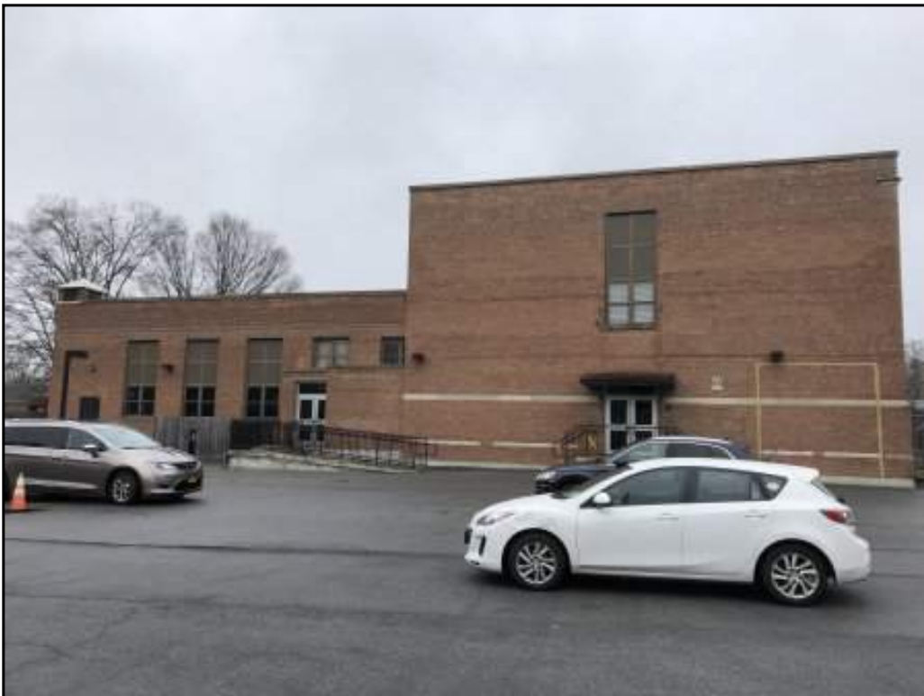
South side of building from parking lot, facing N
