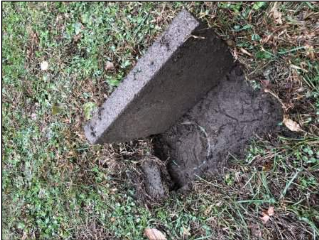
Top of pipe, possible cleanout or access to septic system d-box
