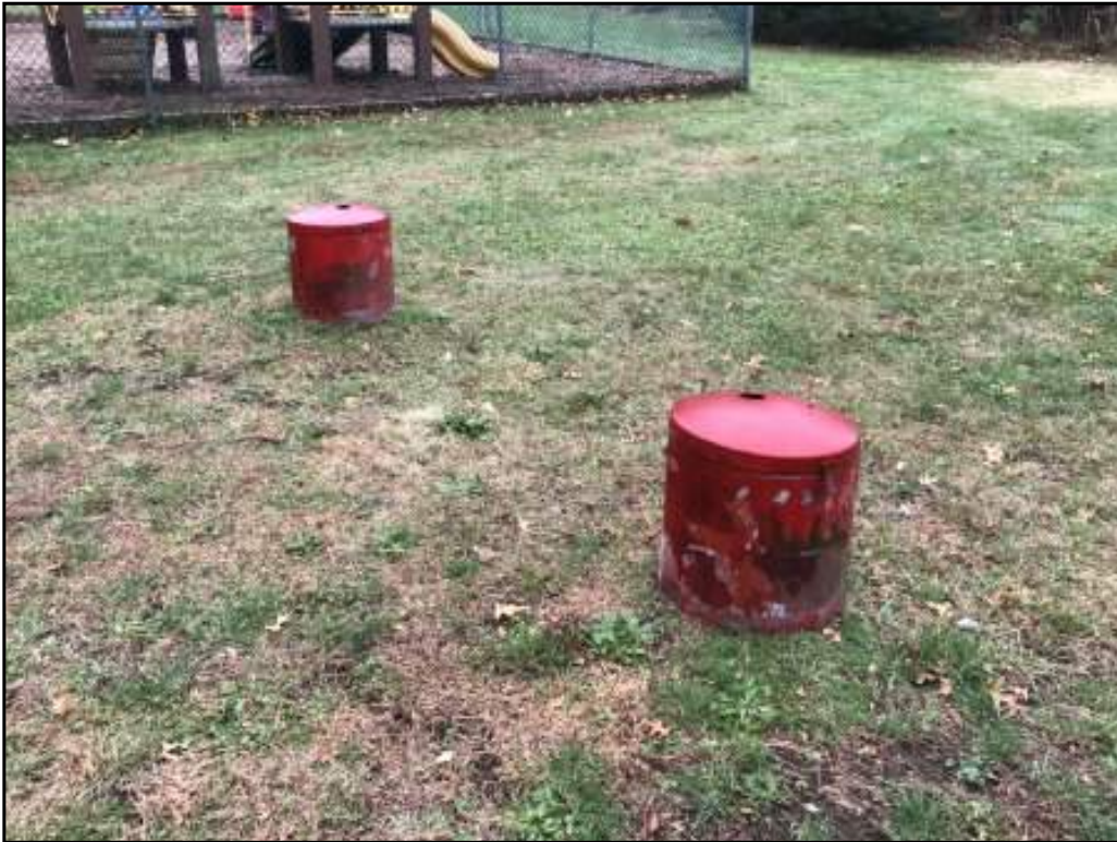
Access to buried propane tank valves NW of building, facing SW
