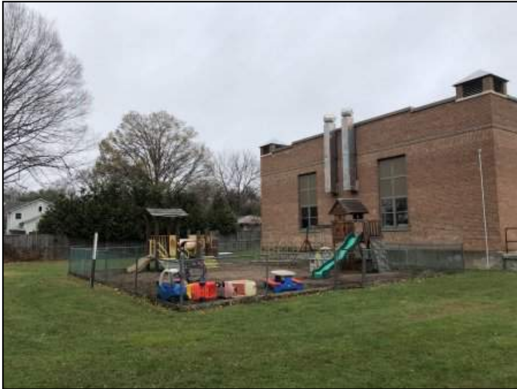
Western side of building, facing NE
