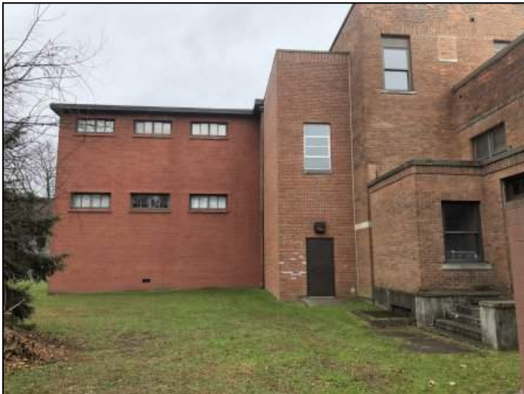
Northern side of building, facing W from NW corner
