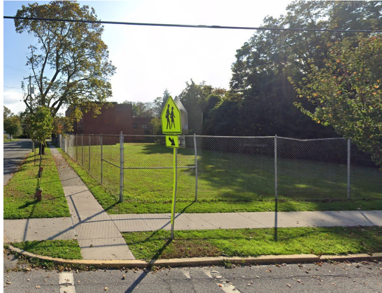
Figure 1. A portion of the existing chain link fence which runs the perimeter of the project property.
